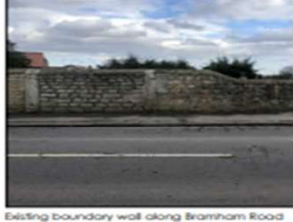
Existing boundary wall along Bramham Road
