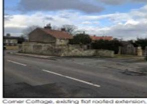
Corner Cottage, existing flat roofed extension, and boundary wall viewed from the southwest
