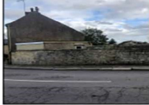
Corner Cottage, existing flat roofed extension wall viewed from the west
